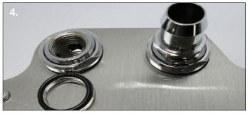
**4.** If you are using G1/4" barbs/fittings with a long thread you will need to use the supplied rings to avoid blocking the flow. Attach the barbs to your chosen ports using an adjustable spanner. Make sure the o-rings are fully compressed.
